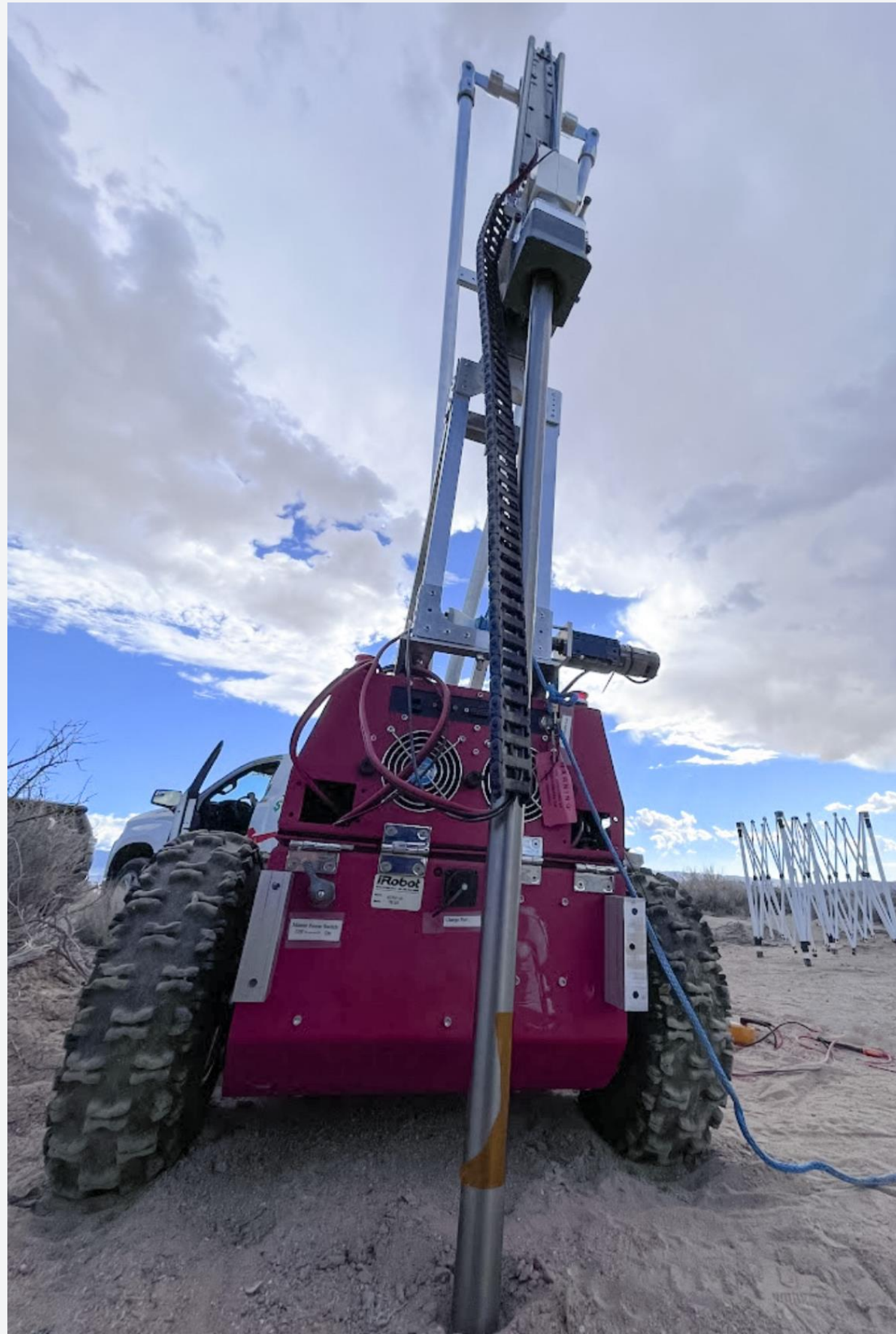
Driving stake into ground
